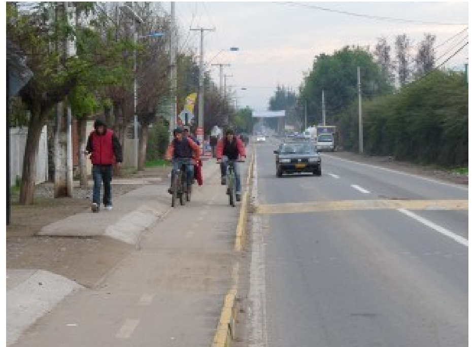
Figure 40: Lack of road safety at road section level. This cycle track is too narrow.
