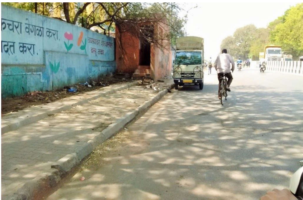
Figure 14: Cyclists being forced to use the carriage way because of unplanned services in the NMT lanes (like public toilets)
