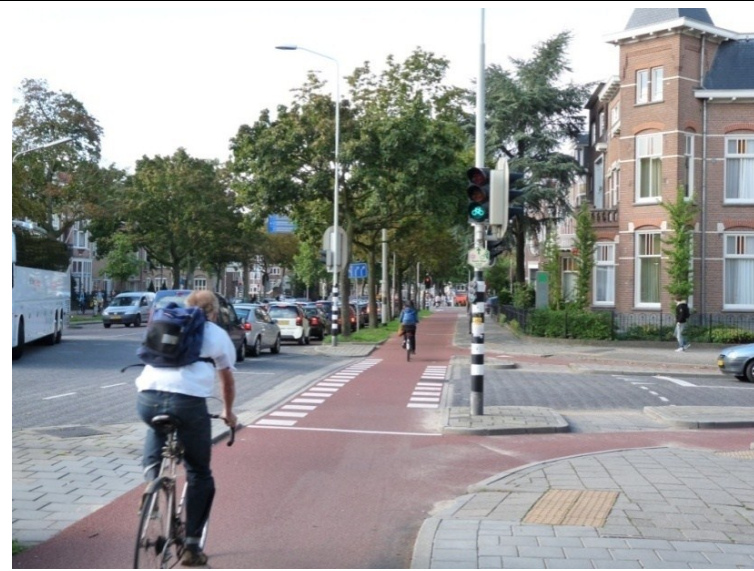
Figure 38: Coherence at intersection level: cycle track is clearly marked across the intersection
