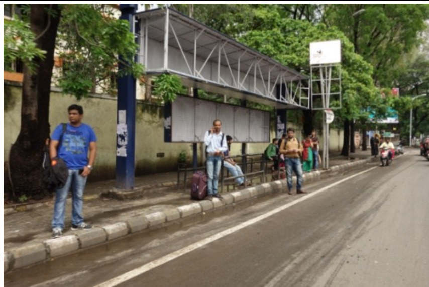
Figure 37: No continuity of cycle track at bus stop (Ganeshkhind Road)
