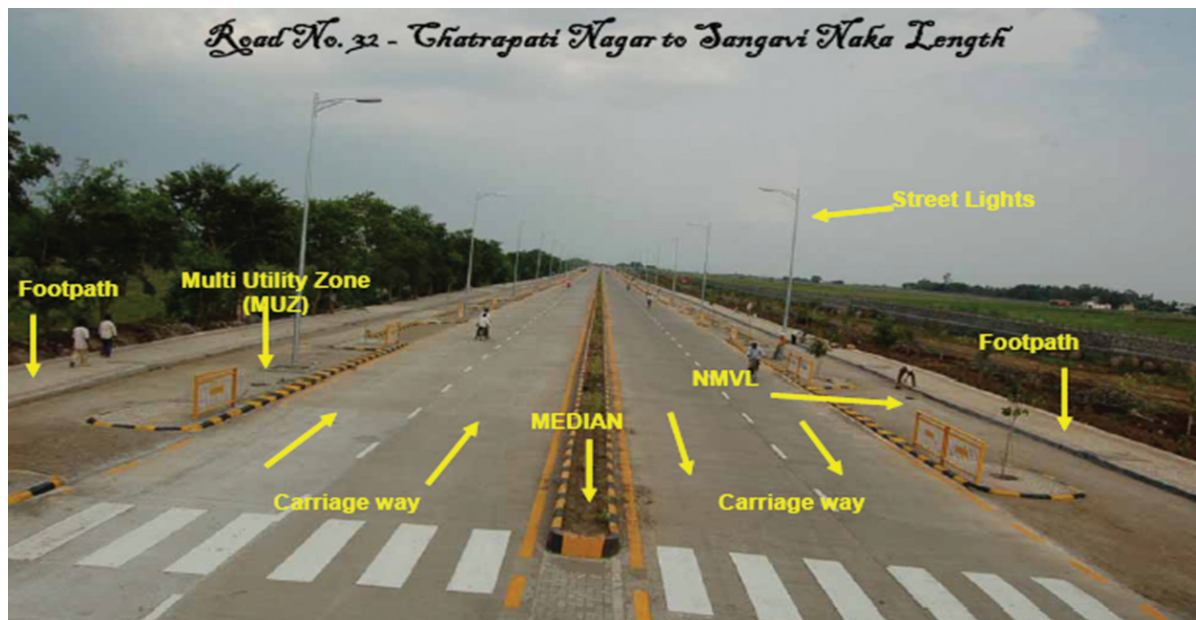
Figure 8: Upgraded streets of Nanded
