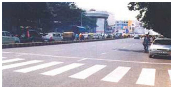
Figure 9: M.G. Road, completed footpath and road
