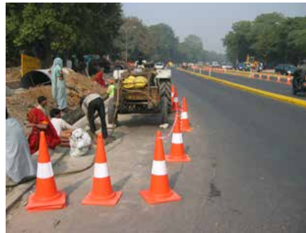
Figure 41 : Use of channelizing devices during construction. (Source: SGArchitects,Delhi)
