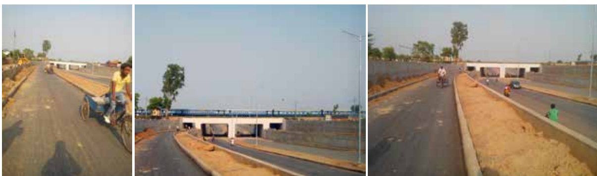
Figure 24: Grade Separated Crossing for NMV (ongoing construction), Chandigarh
