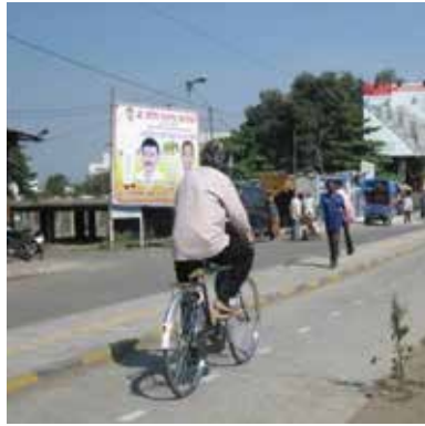
Segregated cycle track on Solapur Road Source :Prasanna Desai Architects
