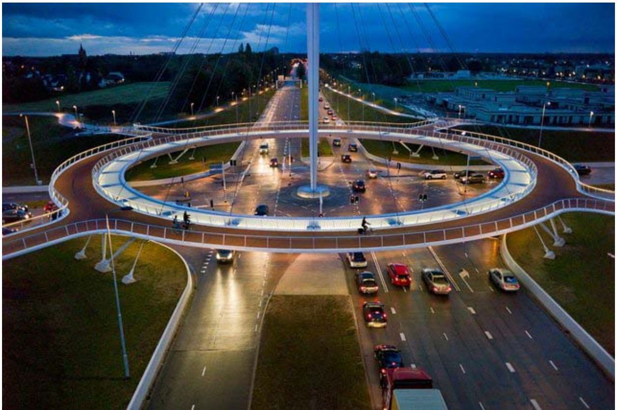
Figure 12: Cycle-only Elevated Roundabout at Intersection in Netherlands
